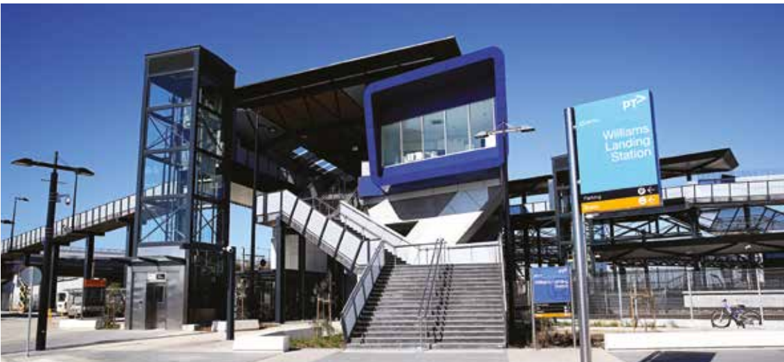
Williams Landing Town Centre, Victoria
