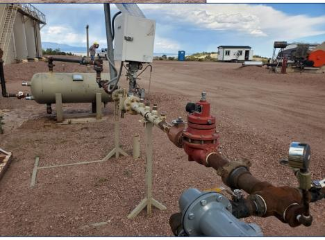
**Figure 3** Gas feed from Pathfinder well to gasfired generators.
