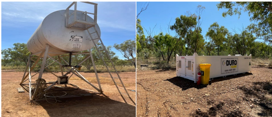
Figure 7: Walford Creek Camp Diesel Fuel Storage (Old and New).
