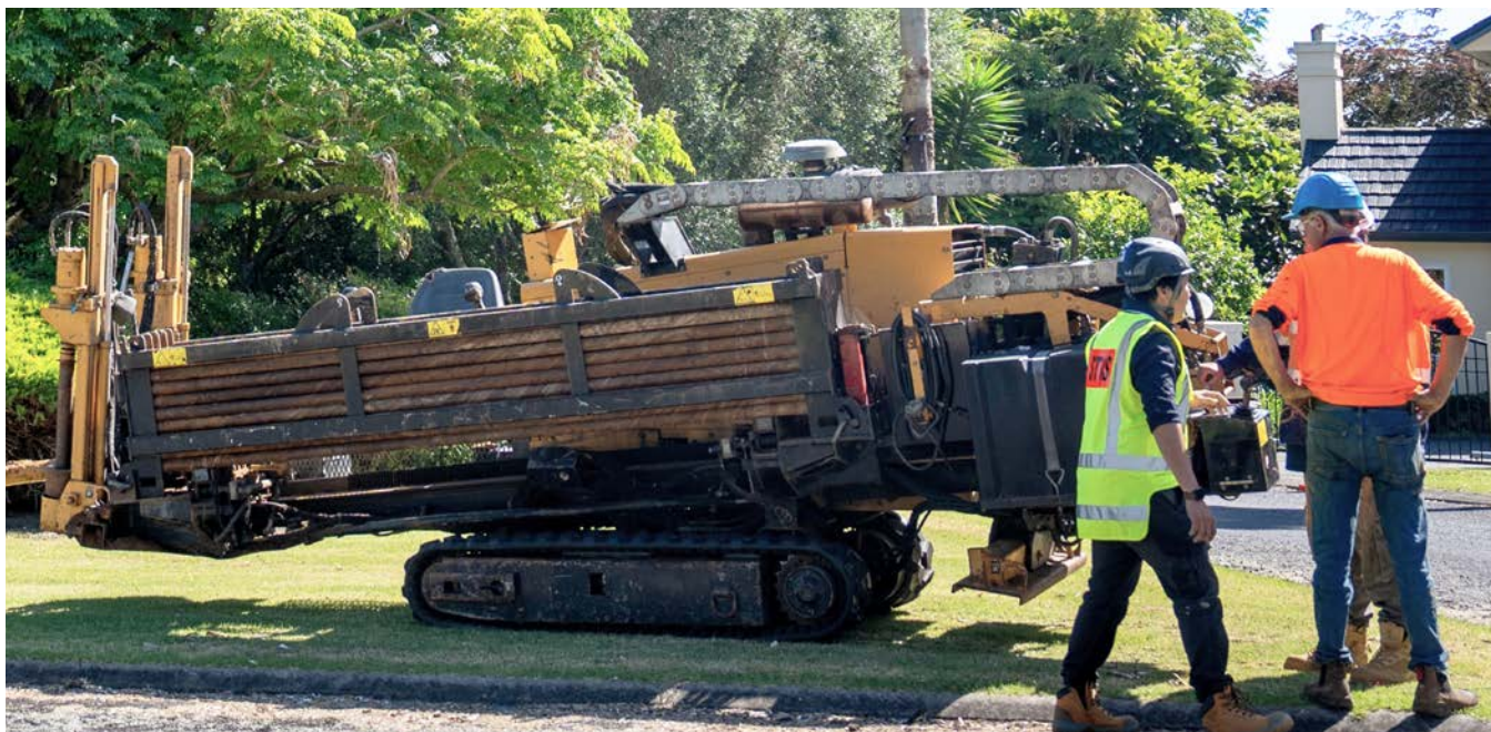
An underground directional drilling machine in Waiau Pa, South Auckland, for the recently announced fibre rollout.
