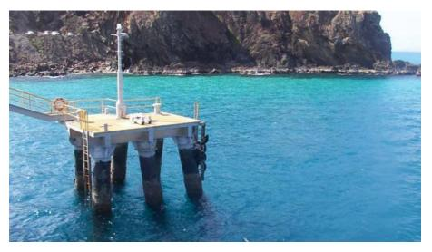
Figure 29: Mooring dolphin structure consisting of 6 raked piles
