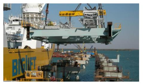
Figure 6: Modulated wharf construction using HLS
