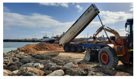
Figure 15: FEL, excavator and dump truck working to place fill for typical armoured rock wharf
