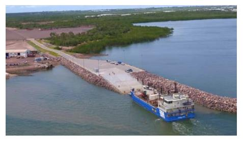
Figure 22: Landing ramp for RORO vessel or landing craft
