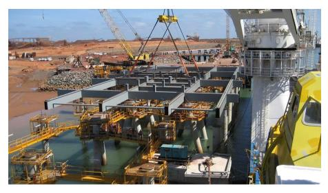
Figure 31: HLS installing prefabricated deck modules
