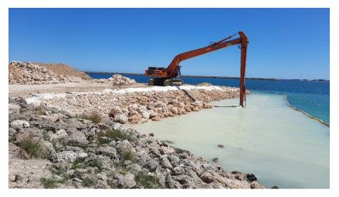
Figure 17: Installation of primary and secondary rock armour on top of geofabric
