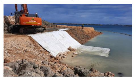
Figure 16: Installation of geofabric on top of fill
