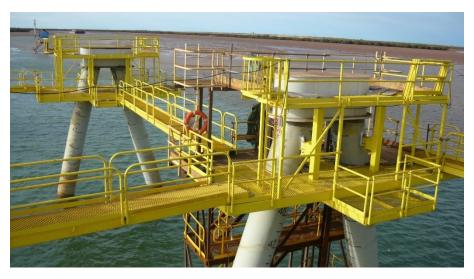
Figure 28: Pile bracing and walkways installed
