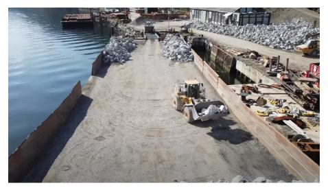
Figure 13: Typical rock barge being loaded by front-end loader
