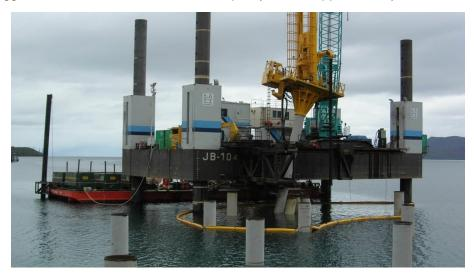
Figure 26: Pile top drill rig and piling frame mounted to SEMP
