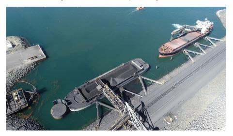
Figure 19: Reference transhipment barge mooring structure
