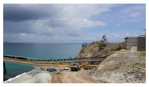
Figure 32: Lack of space on existing conveyor structure for a second conveyor.
