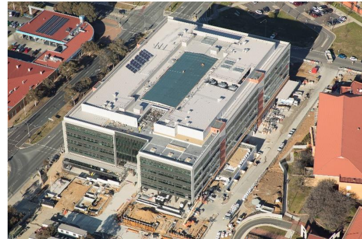
Tuggeranong Building August 2017
