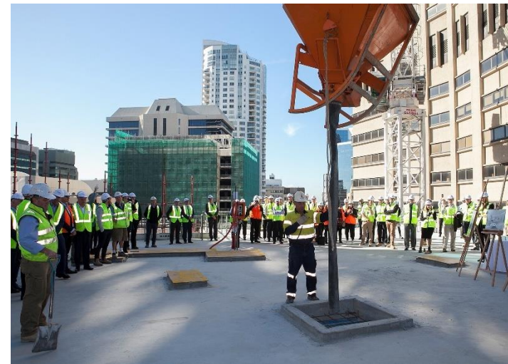
Northpoint Topping Out
