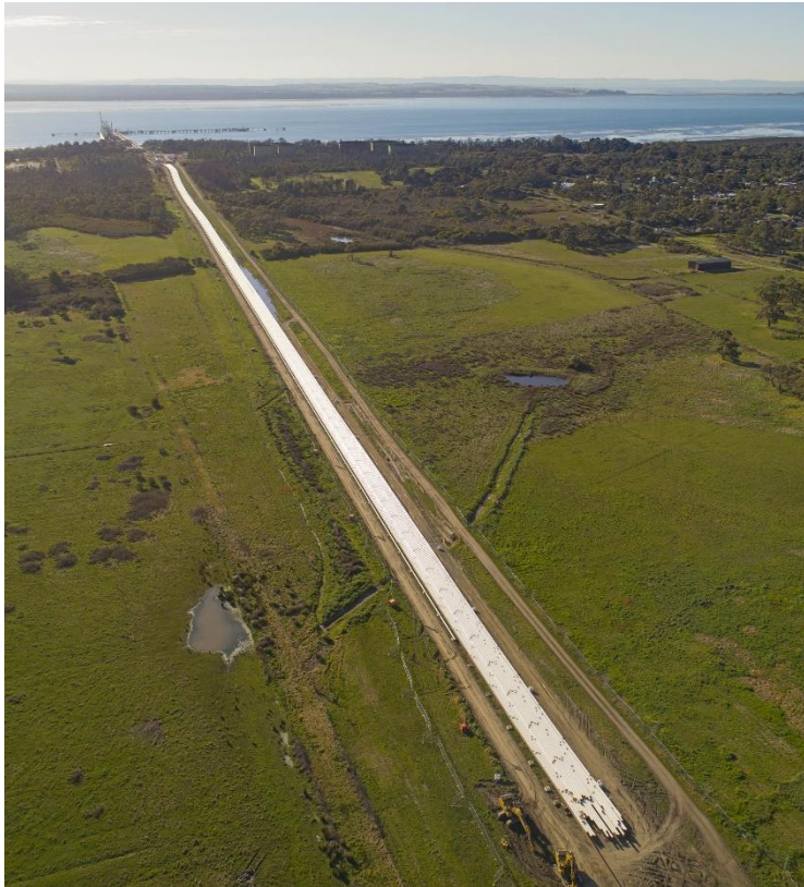
Welded pipe stalks awaiting spooling at Crib Point
