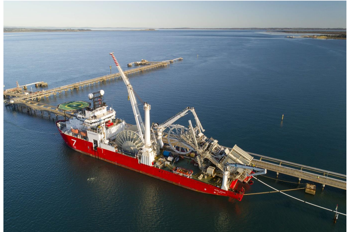
Seven Oceans spooling pipe at Crib Point prior to lay of first section
