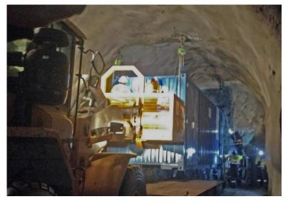
Figure 7: Installation of Primary Fan Motor Control Centre at Syama
