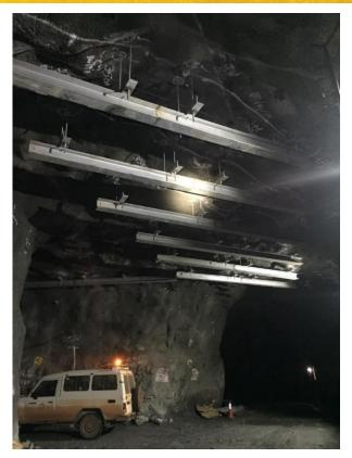
Figure 8: 1105 Pump Station Monorail Installation at Syama
