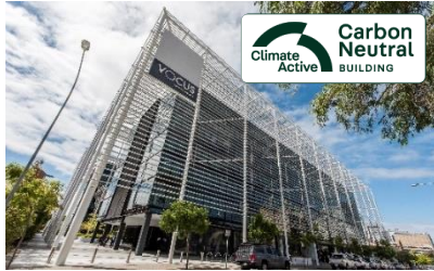
WorkZone West 202 Pier Street, Perth
