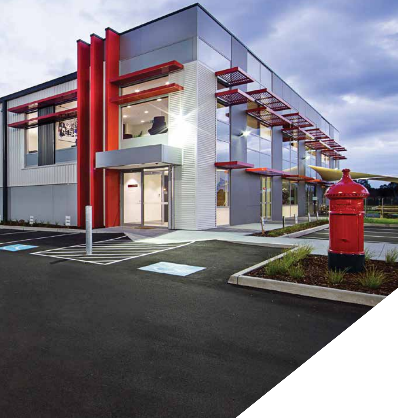
Australia Post, Kingsgrove NSW
