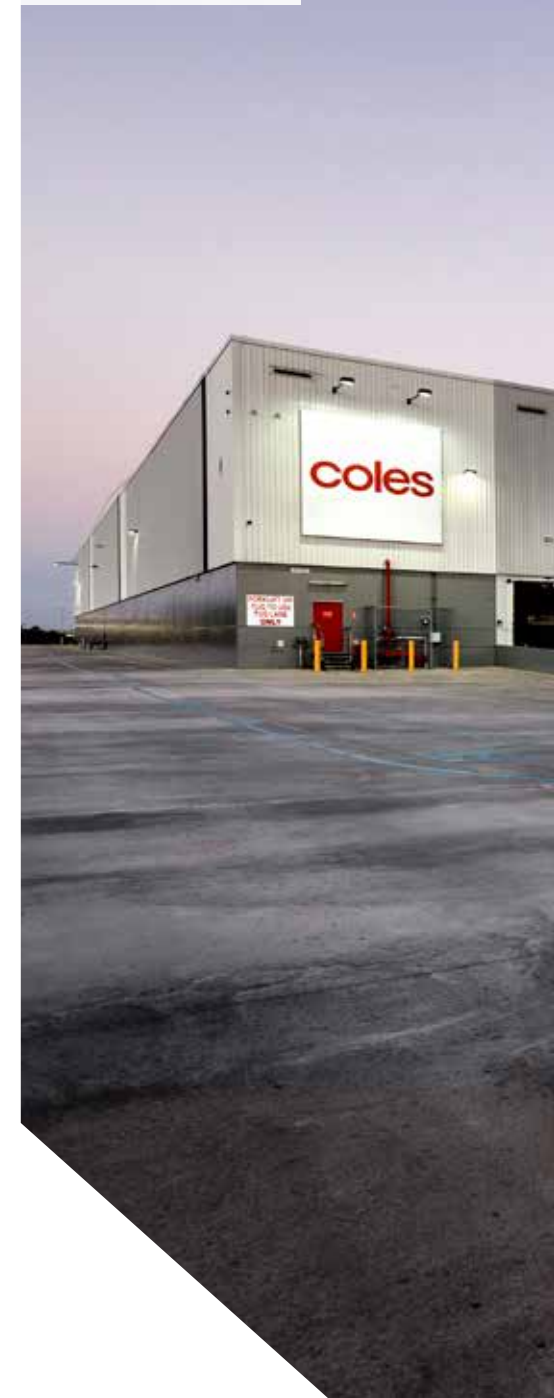
Coles Distribution Centre WA
