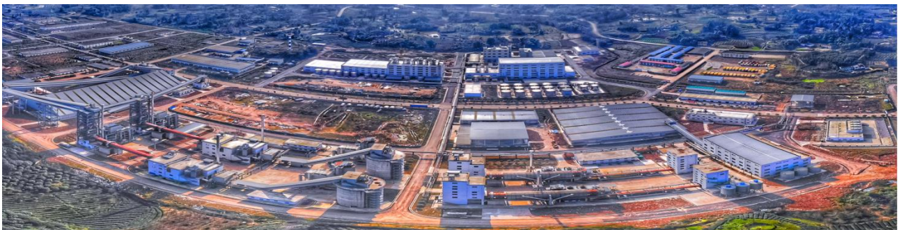
Figure 1: Yahua's 20,000 tonne pa lithium hydroxide plant located in China's southwest province Sichuan
