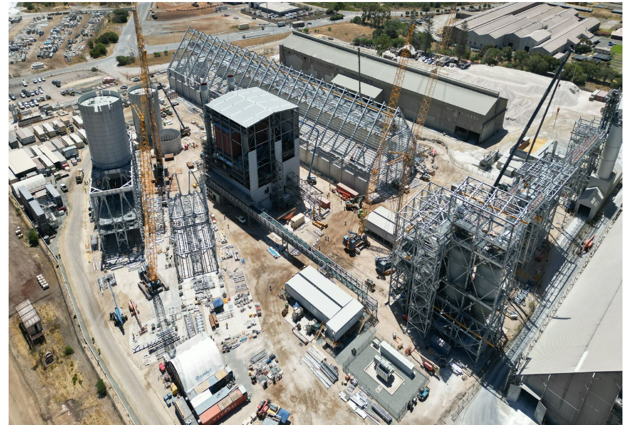
Northern LV Switch-rooms being installed during Q1 2024
