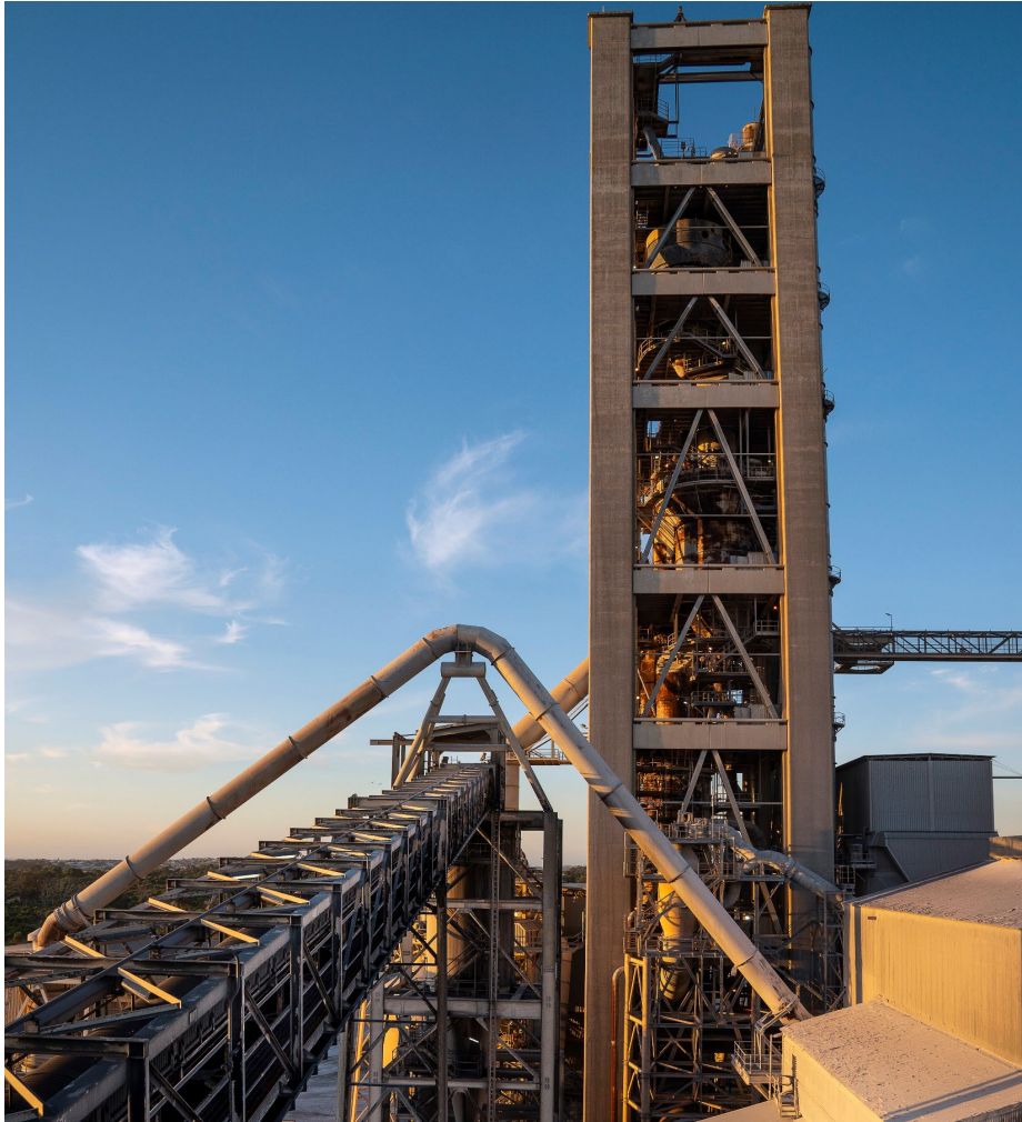
Cockburn Cement Munster lime kiln 6 (pictured) is one of two lime kilns that operate at Munster, with Kiln 5 used primarily to supply Alcoa.
