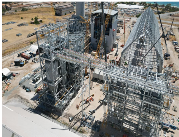
Mill grind and feed building structural works progressing at 72%
