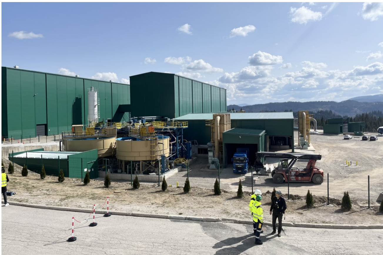
Figure 3: Vares Processing Plant, 5 March 2024
