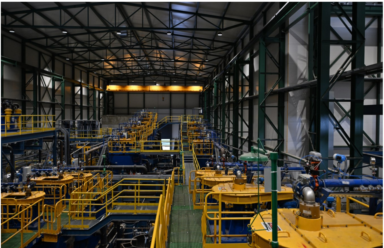
Figure 6: Vares Processing Plant, 5 March 2024
