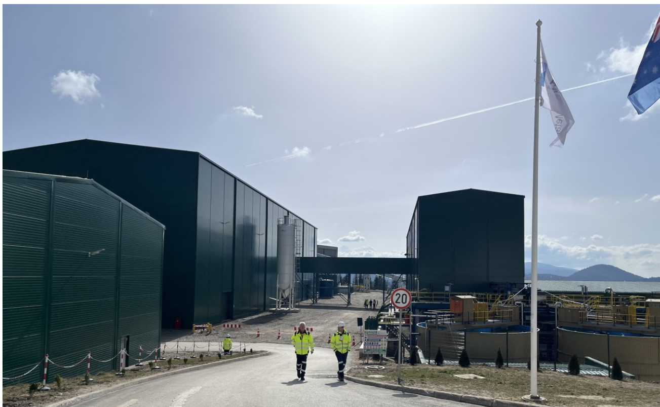
Figure 4: Vares Processing Plant, 5 March 2024
