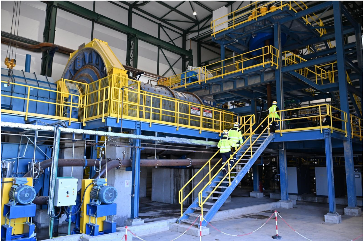
Figure 5: Vares Processing Plant, 5 March 2024
