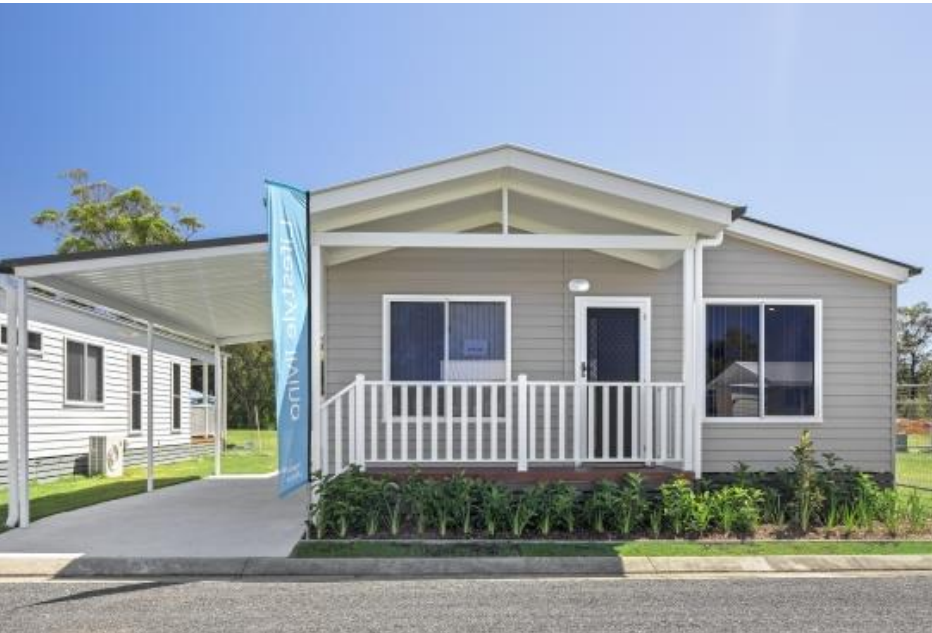
Ingenia South West Rocks, NSW
