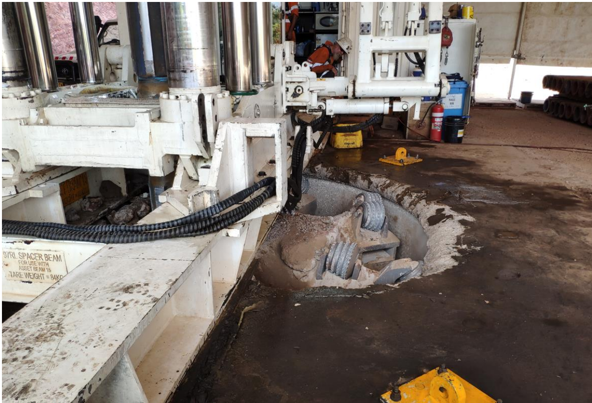
Breakthrough of vent raise at ESS.
