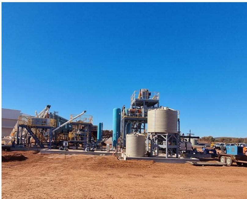
Progress of paste fill plant construction at Golden Grove.
